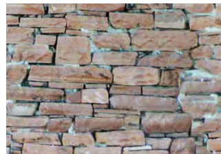
H0 7423 Sandstein Sandstone wall. Grès.
